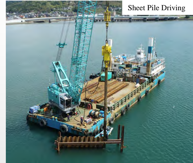
Sheet Pile Driving
