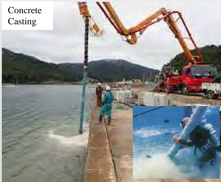
Revetment Construction
