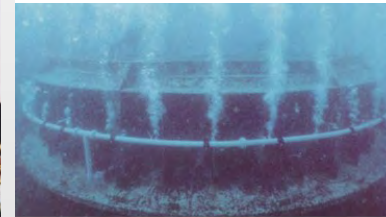
Chlorine Injection Pipeline
